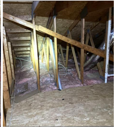
Long attic span with trusses and utilities
