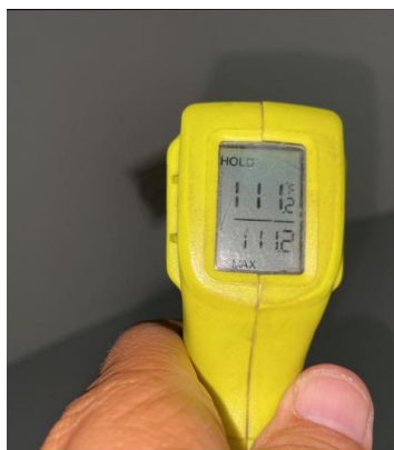
Supply air temperature
