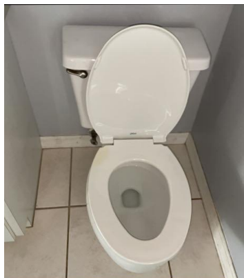
Toilet was loose at the floor at all bathrooms
