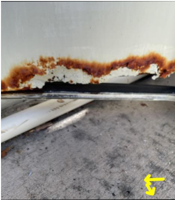
Moisture damage was visible at the door and/or door jamb.
