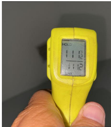
Supply air temperature
