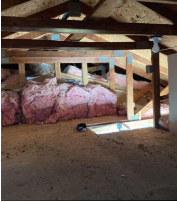
Attic storage space with insulation
