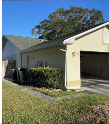
Side view - East
