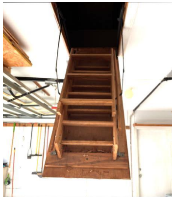
Attic pull down ladder was not fire-rated. (See NACHI Standard of Practice article - https://www.nachi.org/inspectingresidential-attachedgarages.htm ).
