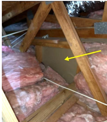
Insulation had been moved/disturbed, leaving low coverage areas
