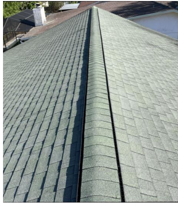
Shingle roof ridge view
