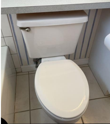
Toilet was loose at the floor at all bathrooms.
