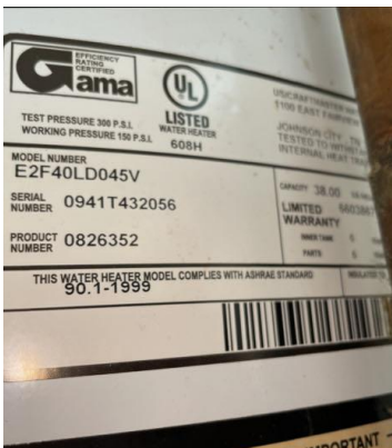
Water heater specification label
