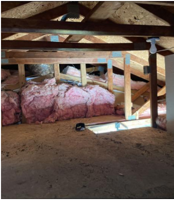
Attic storage space with insulation
