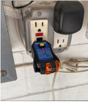
GFCI (Ground Fault Circuit Interrupter) outlet(s) was damaged at garage outlets.
