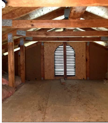
Attic view with gable vent
