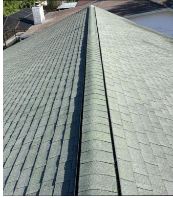
Shingle roof ridge view
