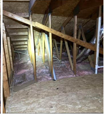
Long attic span with trusses and utilities
