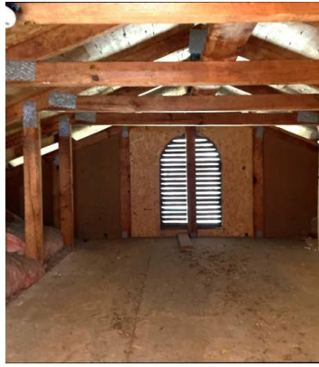
Attic view with gable vent
