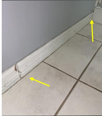
Wall at the exterior of shower enclosure was damaged at the primary bathroom
