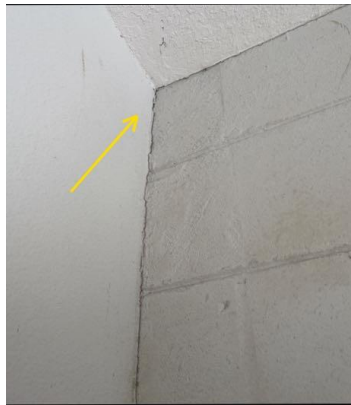
Settlement cracks
