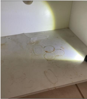
Dry stain(s) were visible under sink at hallway bathroom
